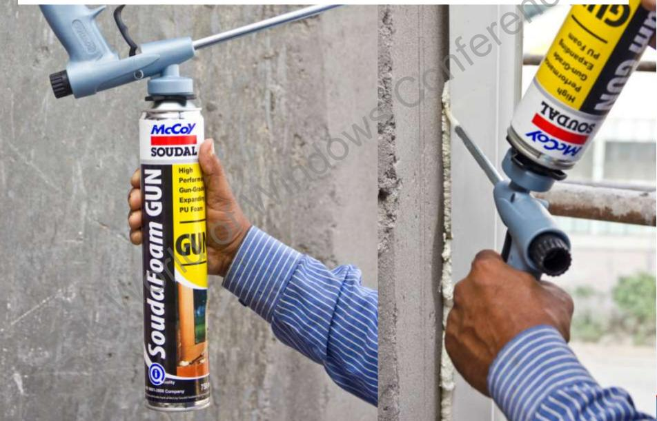
Keep the can always upright during the application. If can is almost empty it will be difficult to extrude the foam if the can is not kept upright
