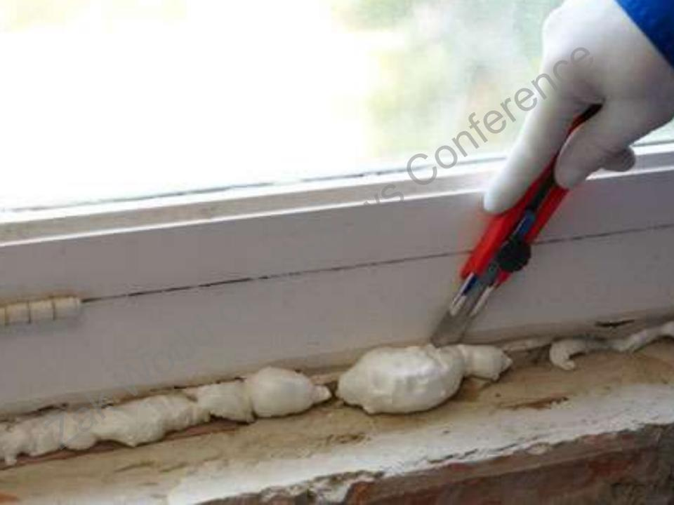
STEP 10: before applying the silicone or acrylic sealant, make sure there is enough depth for the sealant (min. 5mm), if required push the foam deeper into the joint with your finger
